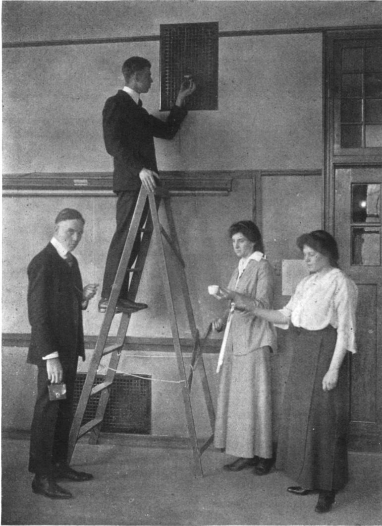
PUPILS USING ANEMOMETER AND SLING-PSYCHROMETER
